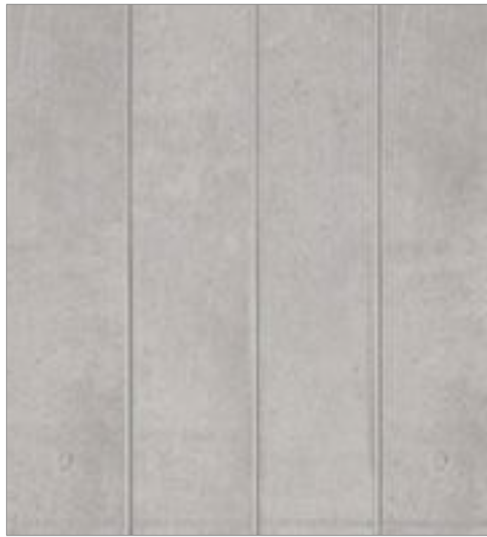
WALLS PRECAST CONCRETE OFF-WHITE MINERAL PAINT FINISH (OR SIMILAR)
